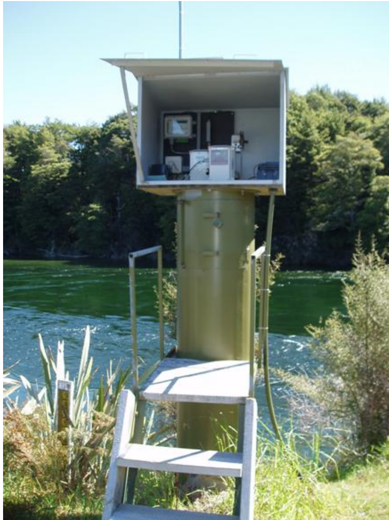
Figure 13 – Typical stilling well housing design.
