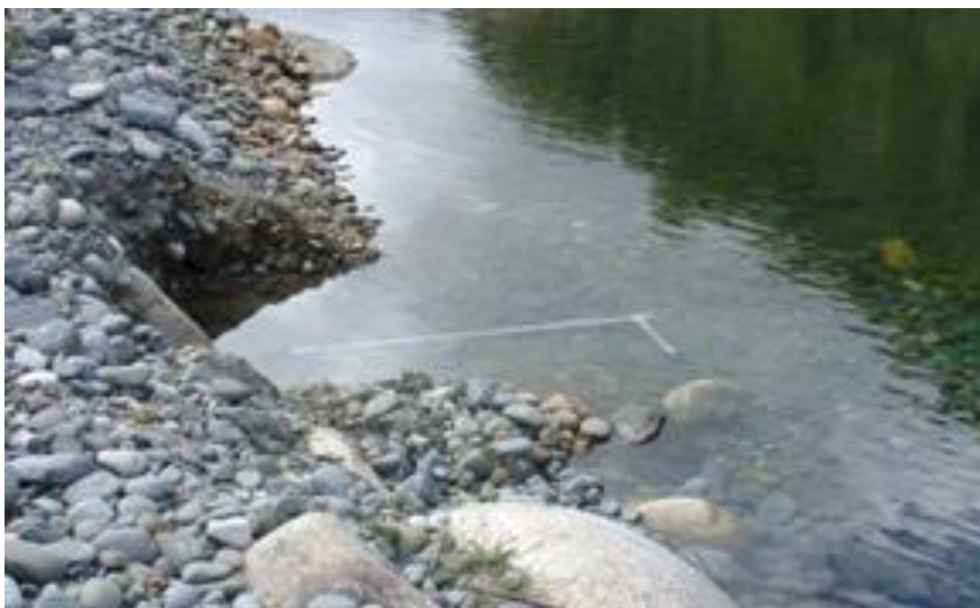
Figure 12 – Example of intake and static pipe.
