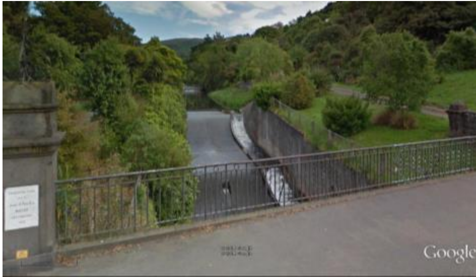
Figure 5 – Leith Stream chute, Dunedin
