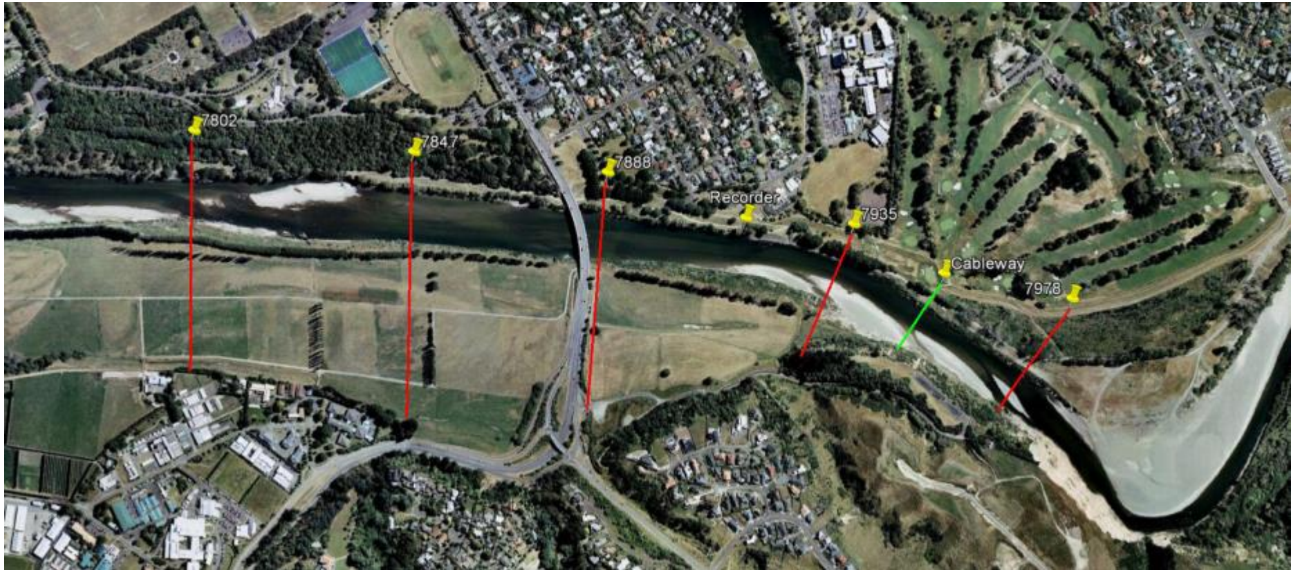
Figure 19 – Recording reach at Manawatu at Teachers College showing location of recorder tower, gauging cableway and surveyed river cross-sections
