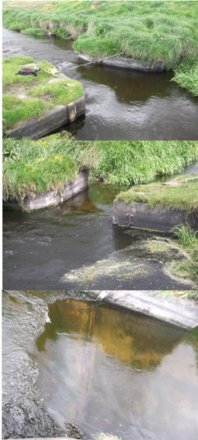
Figure 15 – Awanui Stream Flume Operating Semi-Submerged in the Top and Centre Images, and Under Free-Flow with Formation of a Hydraulic Jump in the Bottom Image
