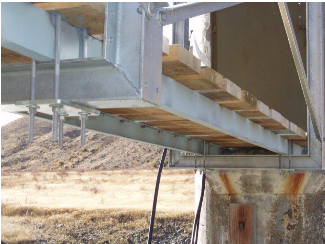
Figure 6 – Underside view of NIWA-design handrail upgrade.
