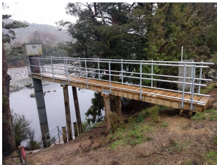
Figure 5 – Timber Catwalk with Steel Handrails
